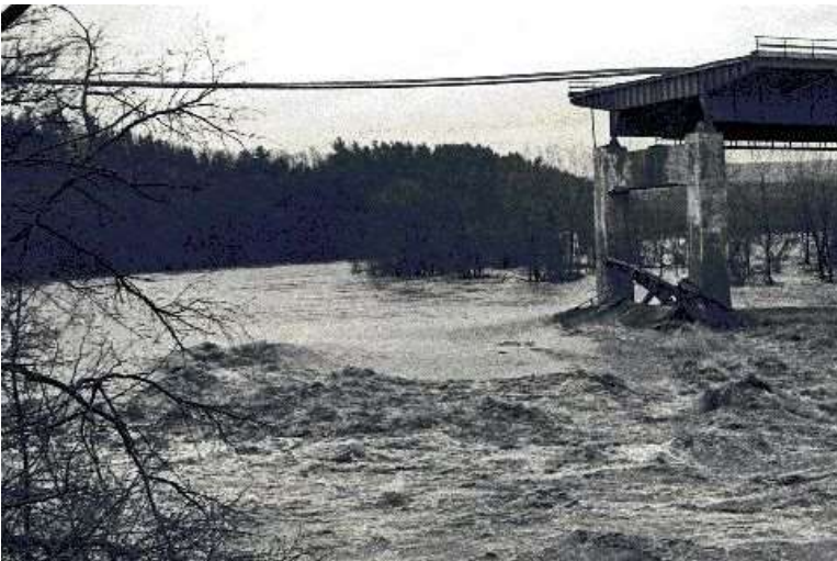
The remains of the I-90 (New York State Thruway) bridge over Schoharie Creek, New York, after a flood undercut the bridge supports and destroyed the bridge. Credit: USGS - http://water.usgs.gov/wid/images/NY.figure.id.3.gif , Public Domain, https://commons.wikimedia.org/w/index.php?curid=56907491
