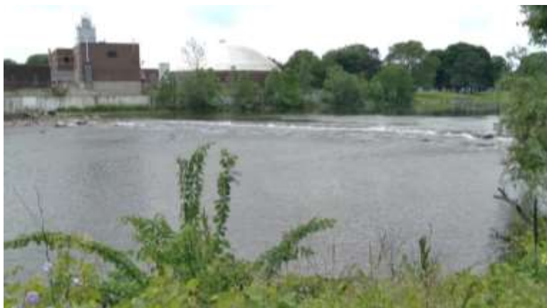
A rock ramp installed just downstream of a small dam on the River Raisin that allows fish to pass. Unfortunately, fish that make it past these modified dams in the city of Monroe are blocked by a still-impassible dam less than 5 miles up from Lake Erie. Credit: Dave Strayer.
