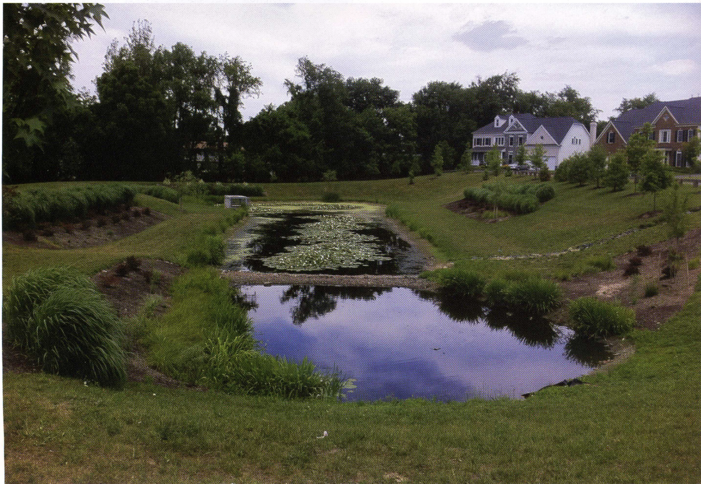
FIG. 5. A stormwater detention pond in a residential suburb of Baltimore (Photo: Chris Swan).
